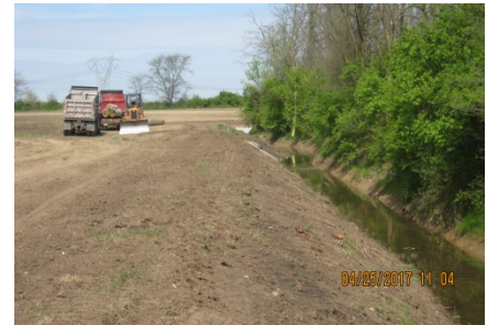
PCE crews cleaning Greenbriar Ext.
