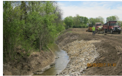
Rock armored curve of Greenbriar Ext.
