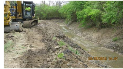
PCE crews cleaning Greenbriar Ext.
