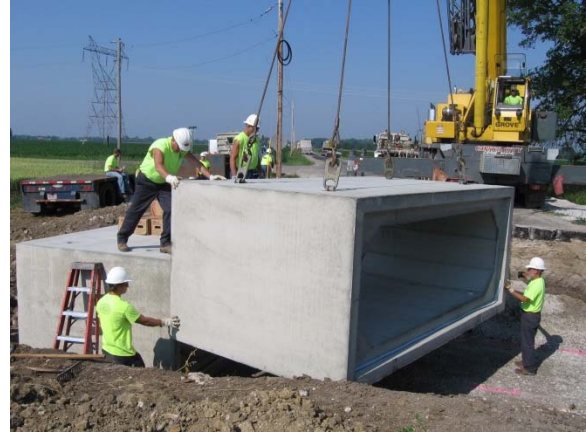
Setting Box Culvert on Whiteside Road
