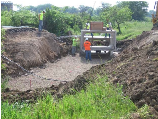
Setting Box culvert on Locust Grove
