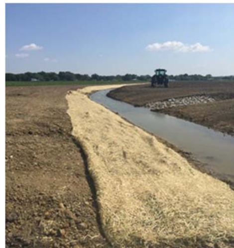
D.S. Drainage Ditch Construction
